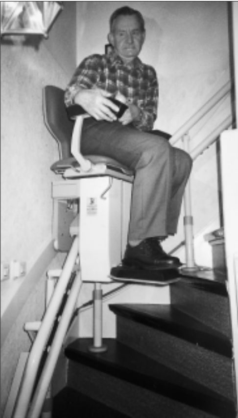
Figure 1: Stairlift in Dutch staircase that is considered too hazardous for use in the United Kingdom
