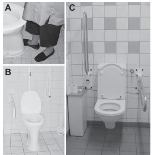
Figure 1. Examples of the toilet bowl as trip object (A), lack of contrast (B), visual balance support (C) and a deceptively continuing floor (C)
