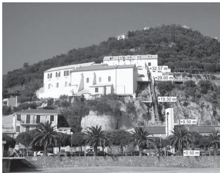
Figure 3 Overview of the renovated Palazzo Vescovile with heights of lift's tops indicated
