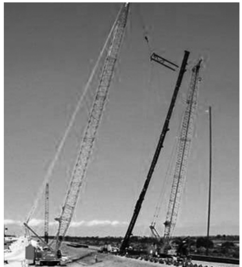
Figure 1. Extreme pile batter with two cranes, template, and swinging leads
